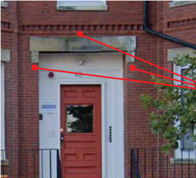
LOCATIONS OF LAG BOLTS INTO BRICK ONLY (NOT CEMENT)
